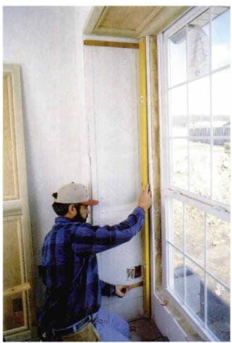
It's a rare house that is perfectly plumb and level. Shims make for a plumb and square nailing surface, and to ease placement, the author builds the floor-to-ceiling panels slightly short, hiding the gap with base molding.
