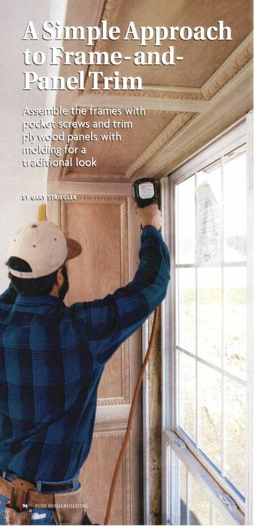
ith my partner, Dan Cobb, I build custom houses in Arkansas. Traditional detailing remains in demand here, and paneled walls are one way I accommodate clients. Because of the cost, I avoid raised panels, instead site-building flat panels from 1/4-in. birch plywood and 4/4 poplar rails (horizontal members) and stiles (vertical members), trimmed with stock moldings. Flat panels lend themselves to applications
